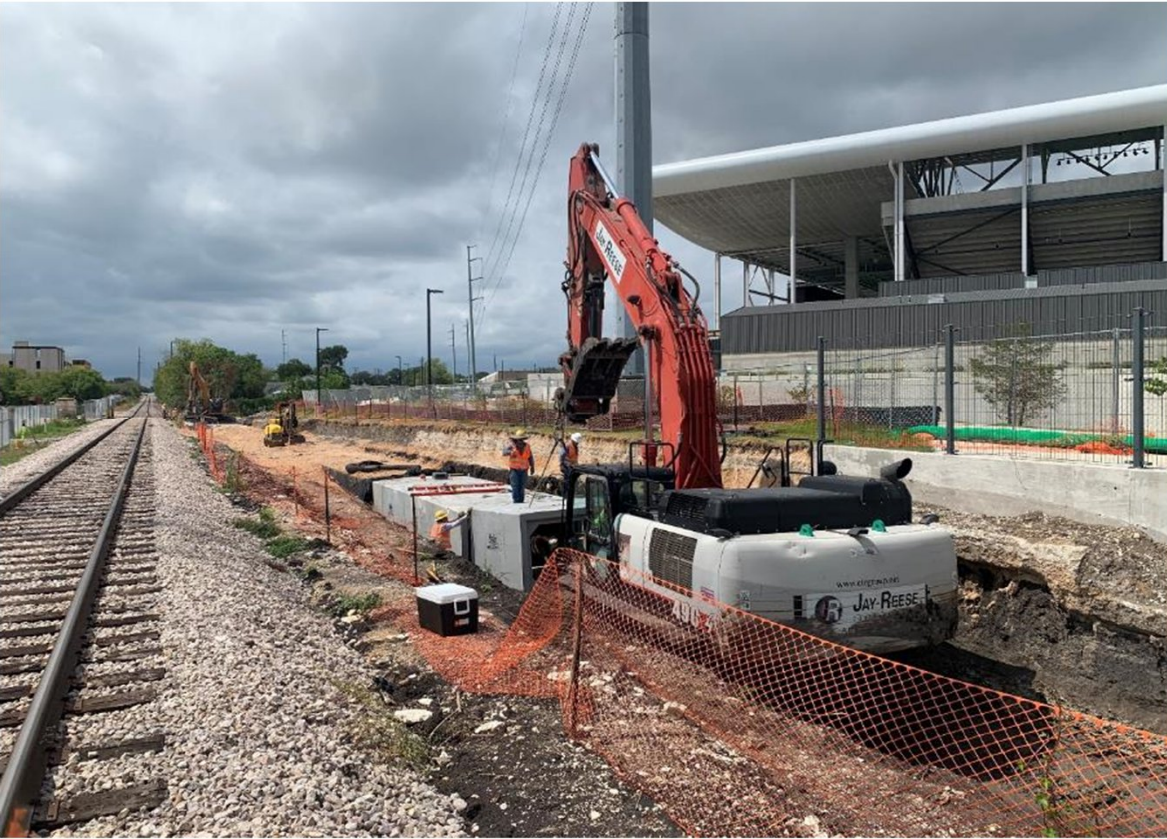
Main Culvert Install
