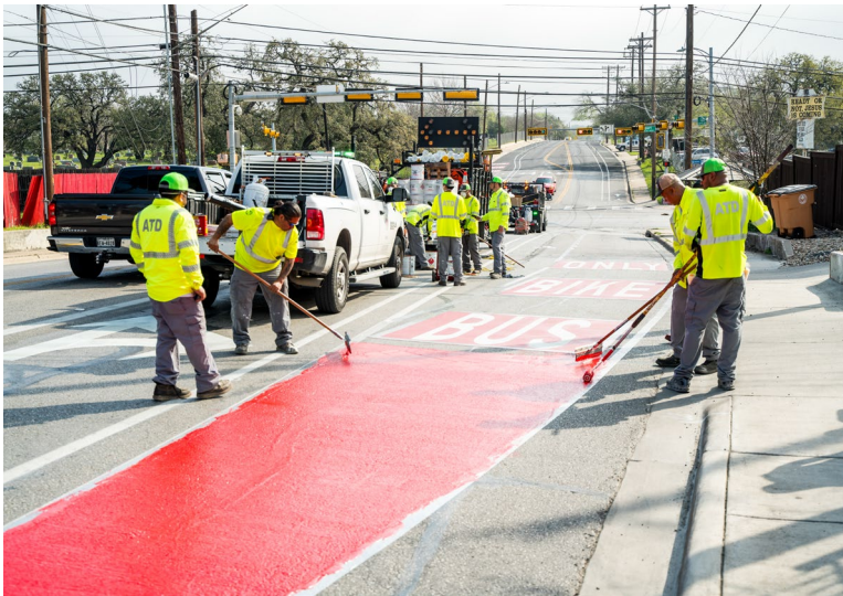
E 12 th at Airport
